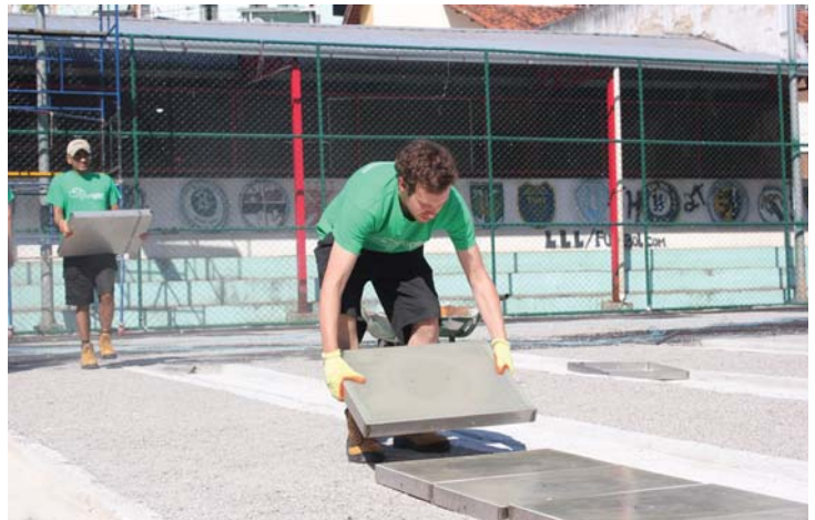
Piezoelectric tiles convert pressure and vibration from people walking on them into electricity to light walkways and fields. (Credit: Pavegen Systems)
